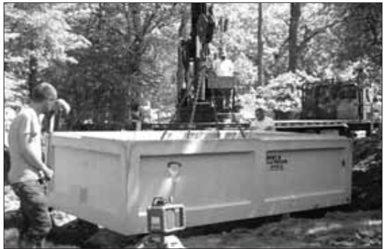
The Bonomos’ tank holds 5,500 gallons of rainwater.
