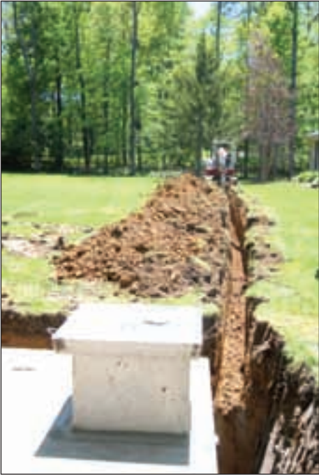
Installation of the system included the digging of trenches for pipelines.
